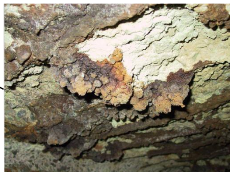
Biogenic sulphuric acid corrosion of concrete – aggressive, fast proceeding decrease .
